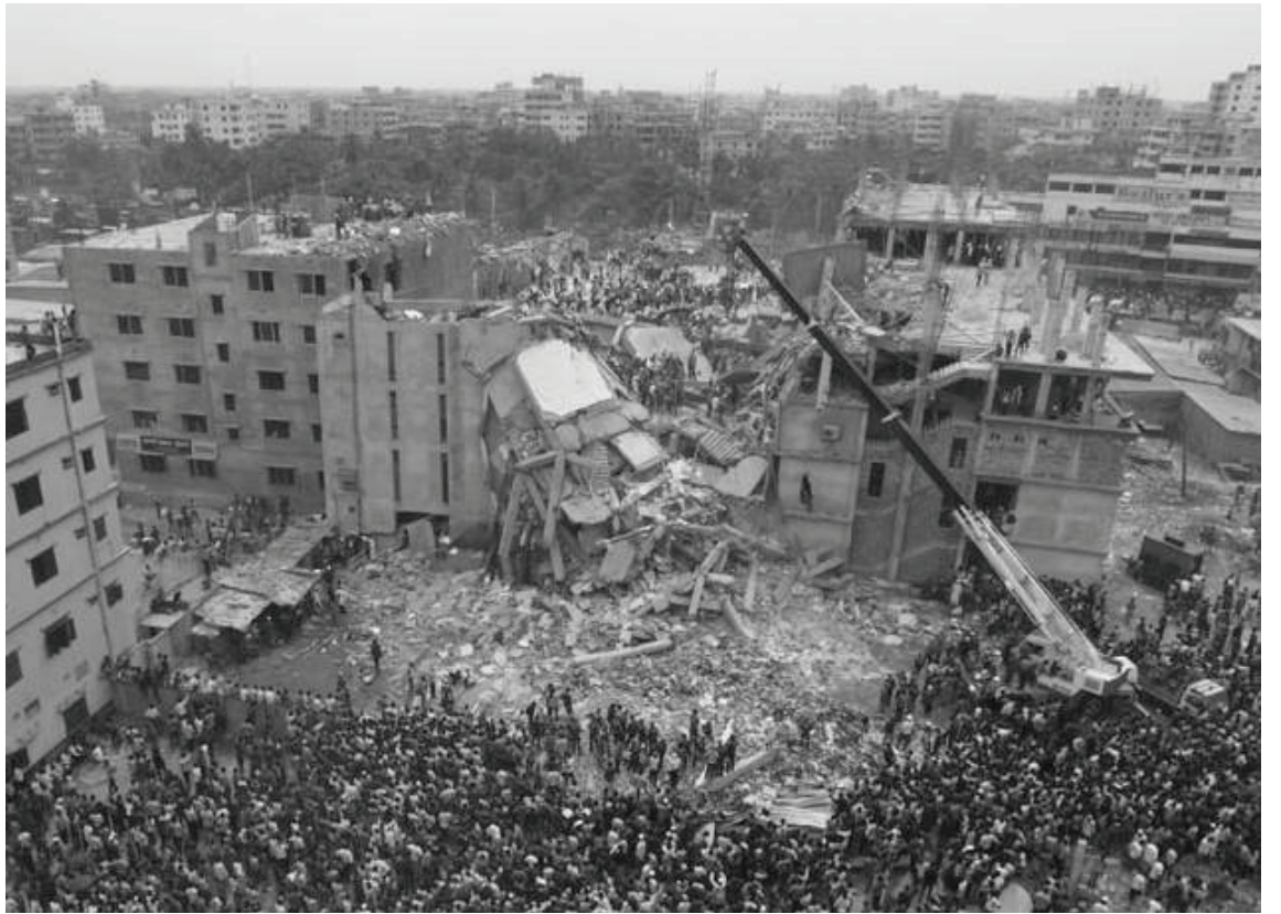
An aerial view of the collapse in Savar, Bangladesh. Photo Credit: libcom.org
